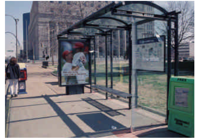
Bus shelter. St. Louis, MO.
