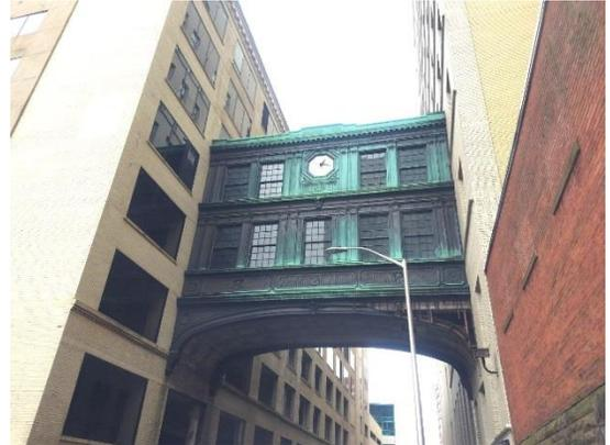
The copper-clad pedestrian bridge was built to connect the G. Fox and Company department store to its warehouse building on Talcott Street.
