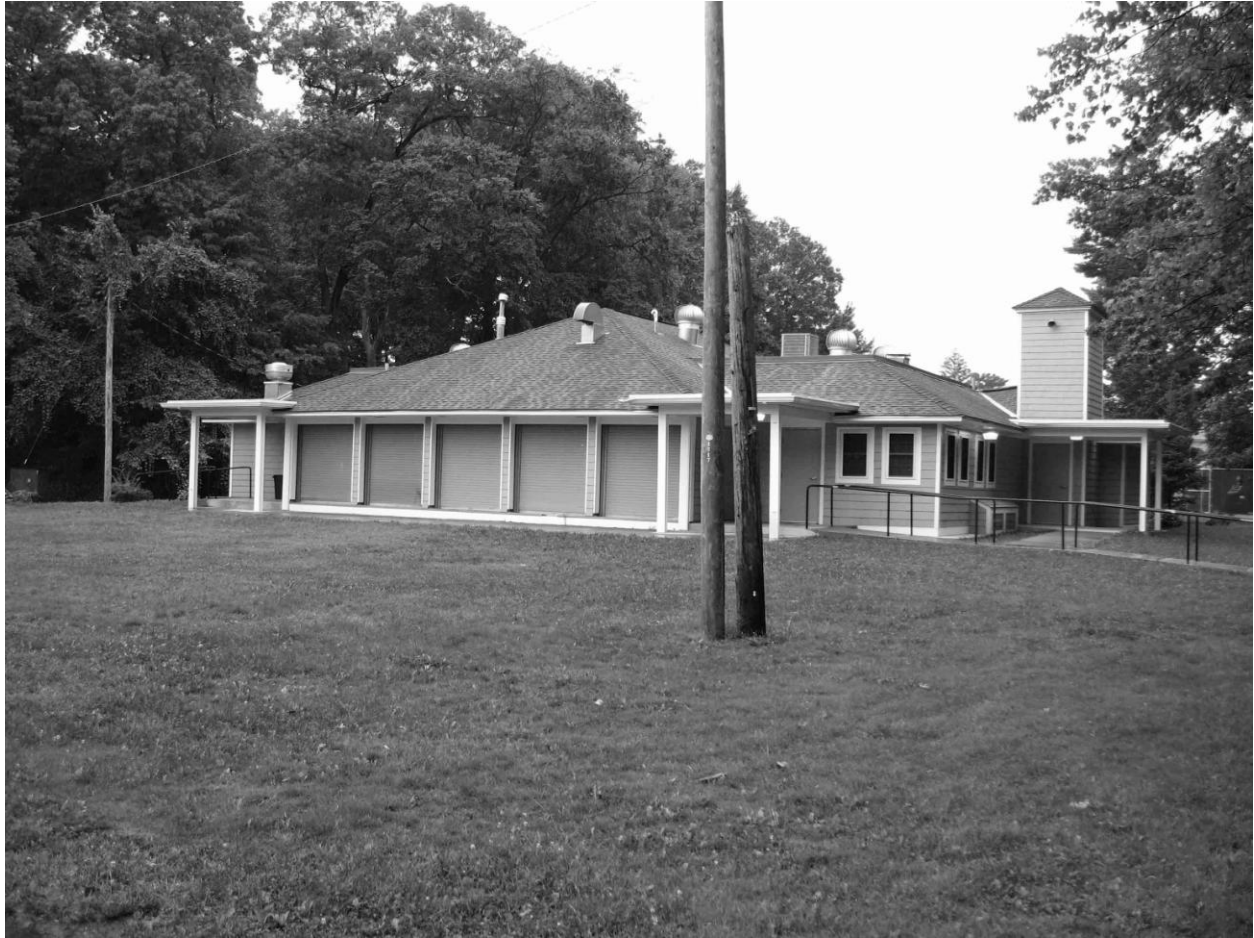
Photograph 7 of 38 Rear of Keney Park pond house (323 Edgewood Street) Camera facing northeast
