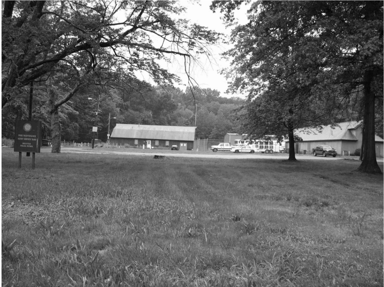
Photograph 16 of 38 Ebony Horsewomen and Hartford Mounted Patrol stables and maintenance barns Camera facing west
