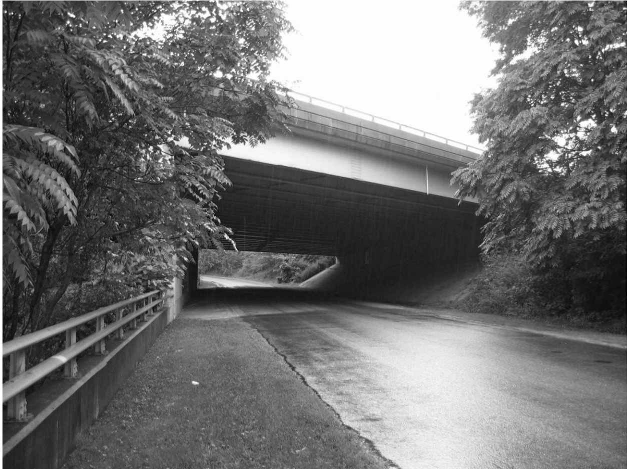
Photograph 31 of 38 US Interstate 91 bridge traversing park road Camera facing west
