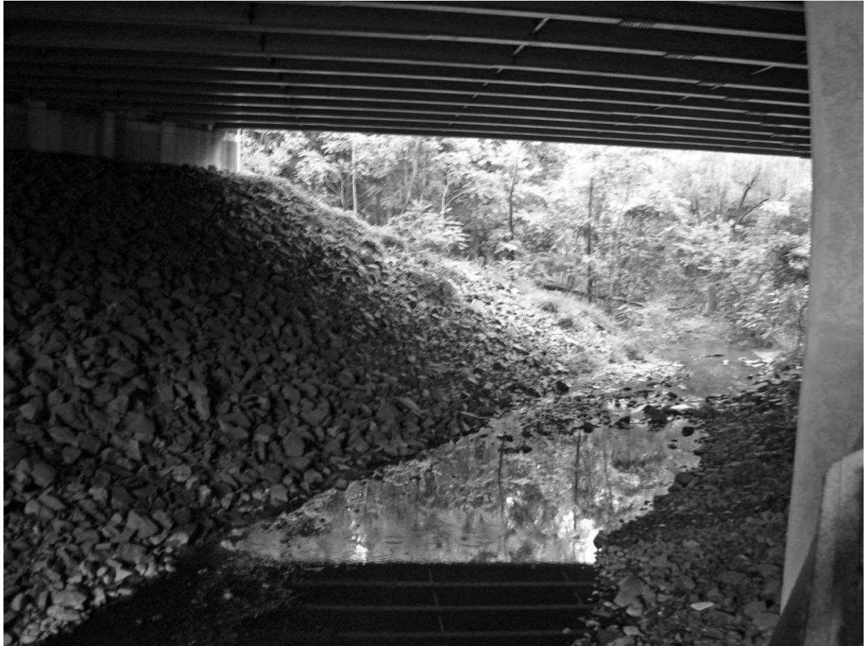
Photograph 37 of 38 Midvale Stream and portion of the Gorge under the US Interstate 91 bridge in East Open Camera facing west
