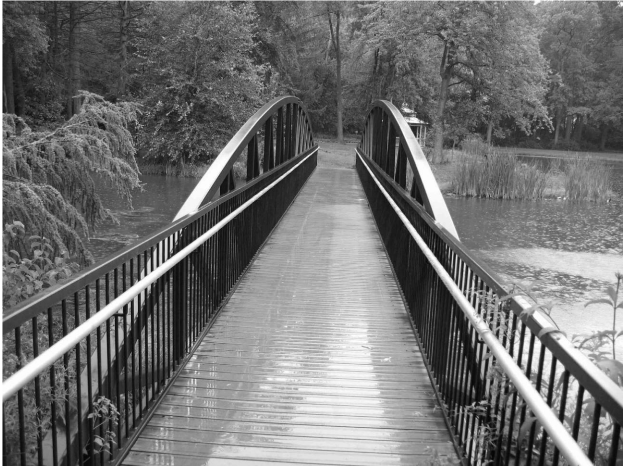
Photograph 11 of 38 Footbridge over the pond Camera facing east
