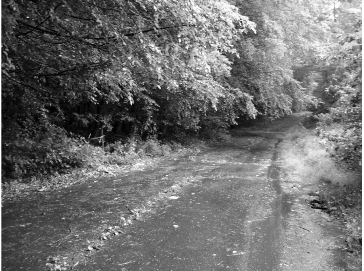
Photograph 18 of 38 Currently unused roadway through Bushland Camera facing north
