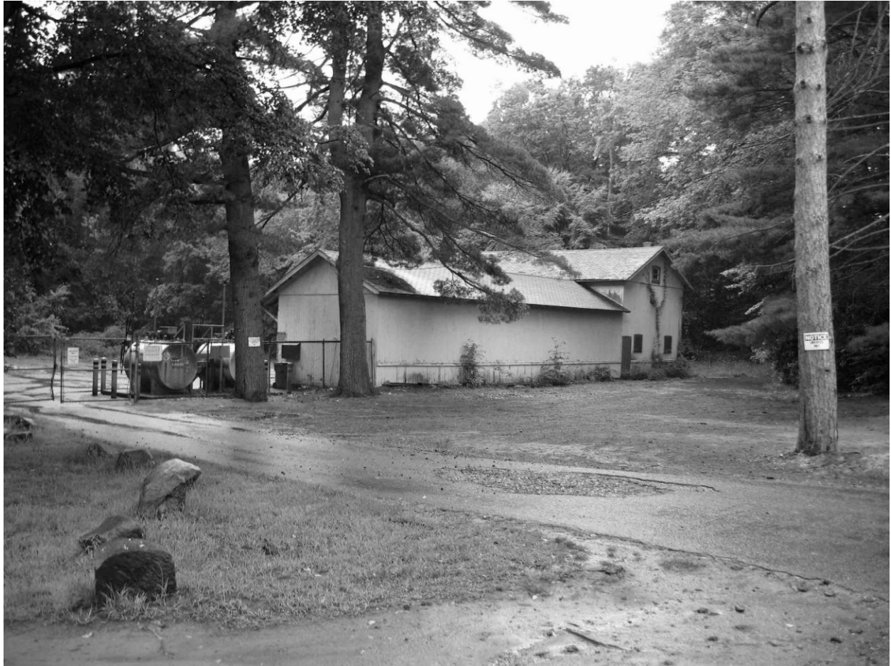
Photograph 22 of 38 Golf course maintenance barn Camera facing southwest
