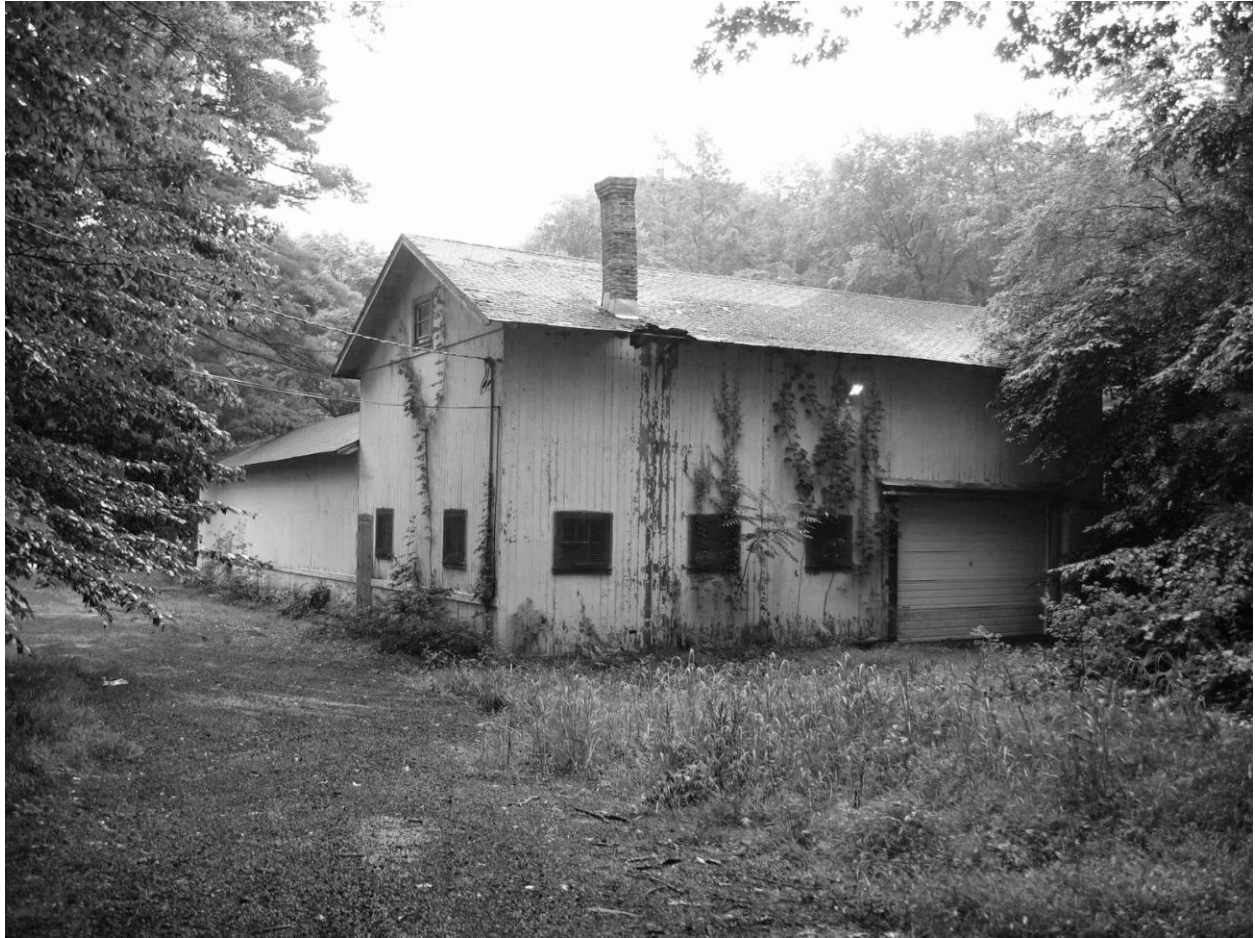
Photograph 23 of 38 Golf course maintenance barn Camera facing east
