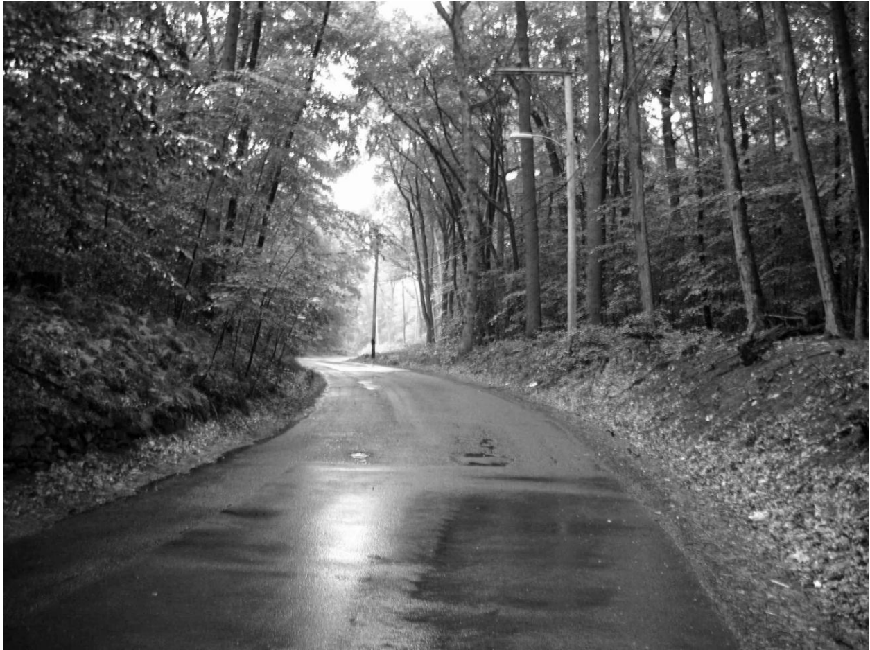
Photograph 29 of 38 Park roadway in Ten Mile Woods section; note built-up mounds on either side of road, a design feature intentioned by the Olmsteds Camera facing north
