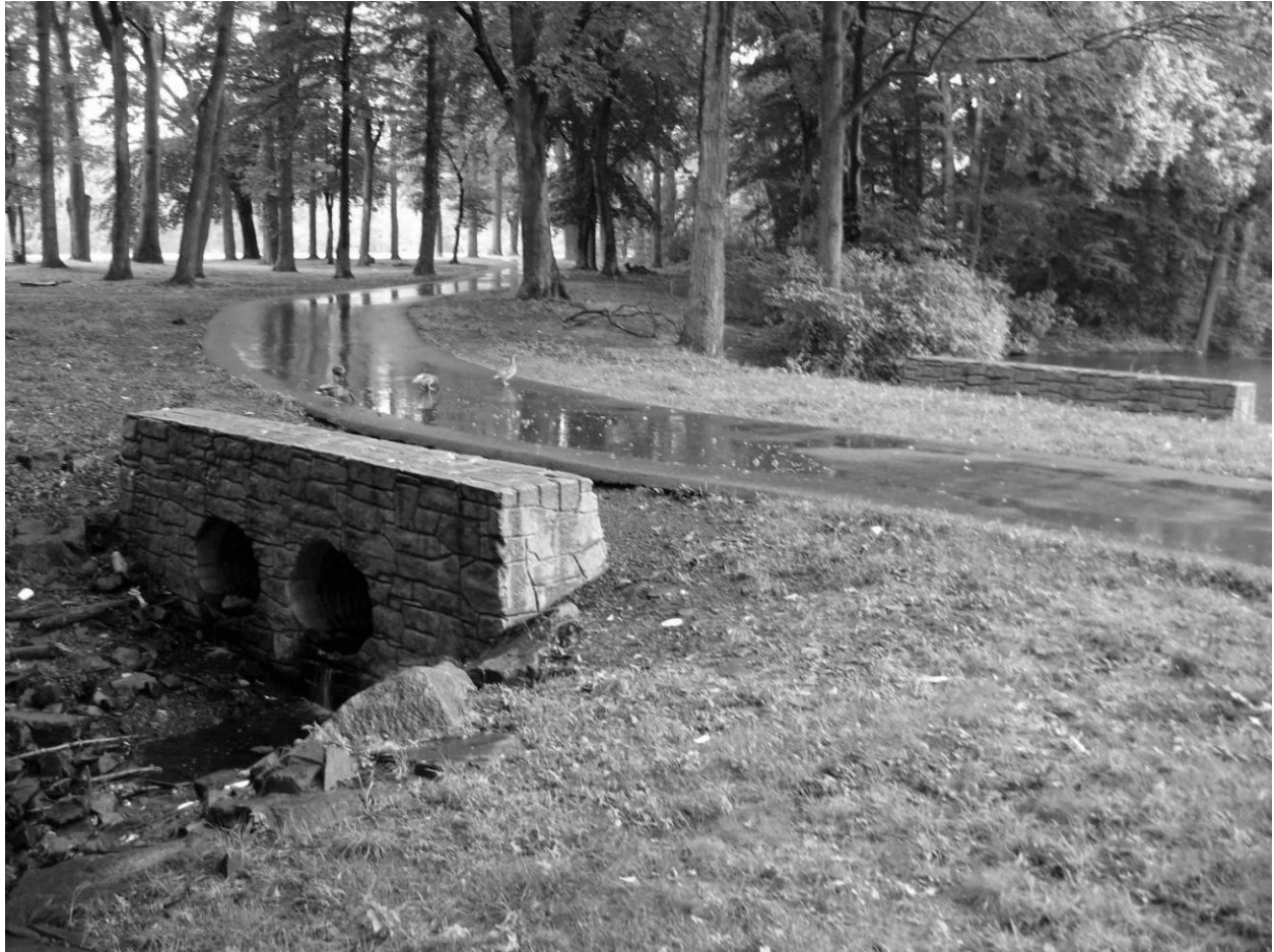
Photograph 14 of 38 Footbridge in West Open over tributary of the pond Camera facing west
