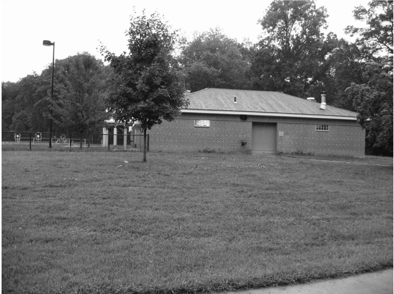
Photograph 6 of 38 Keney Park pool house in the West Open Camera facing north
