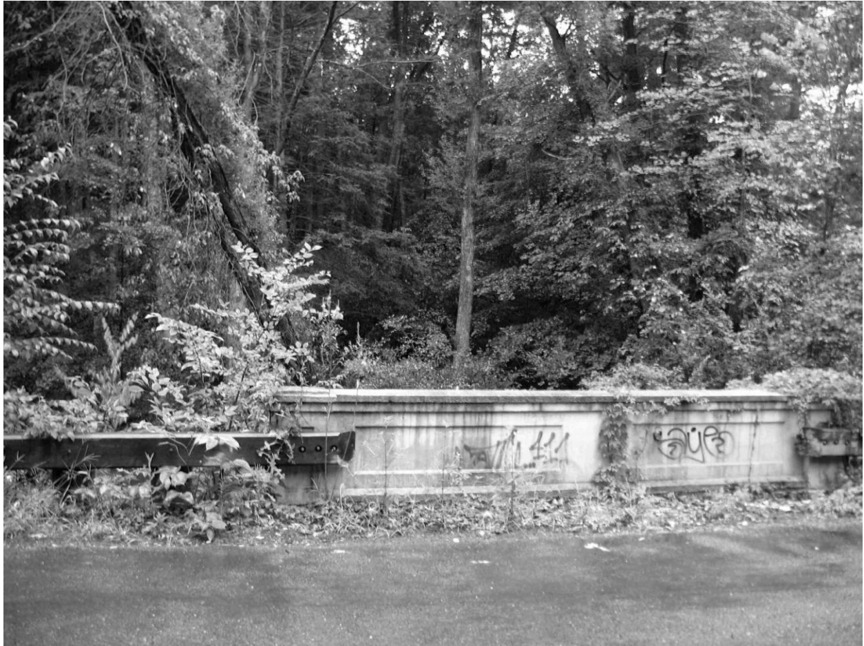
Photograph 30 of 38 Concrete bridge in East Open traversing Midvale Stream Camera facing north
