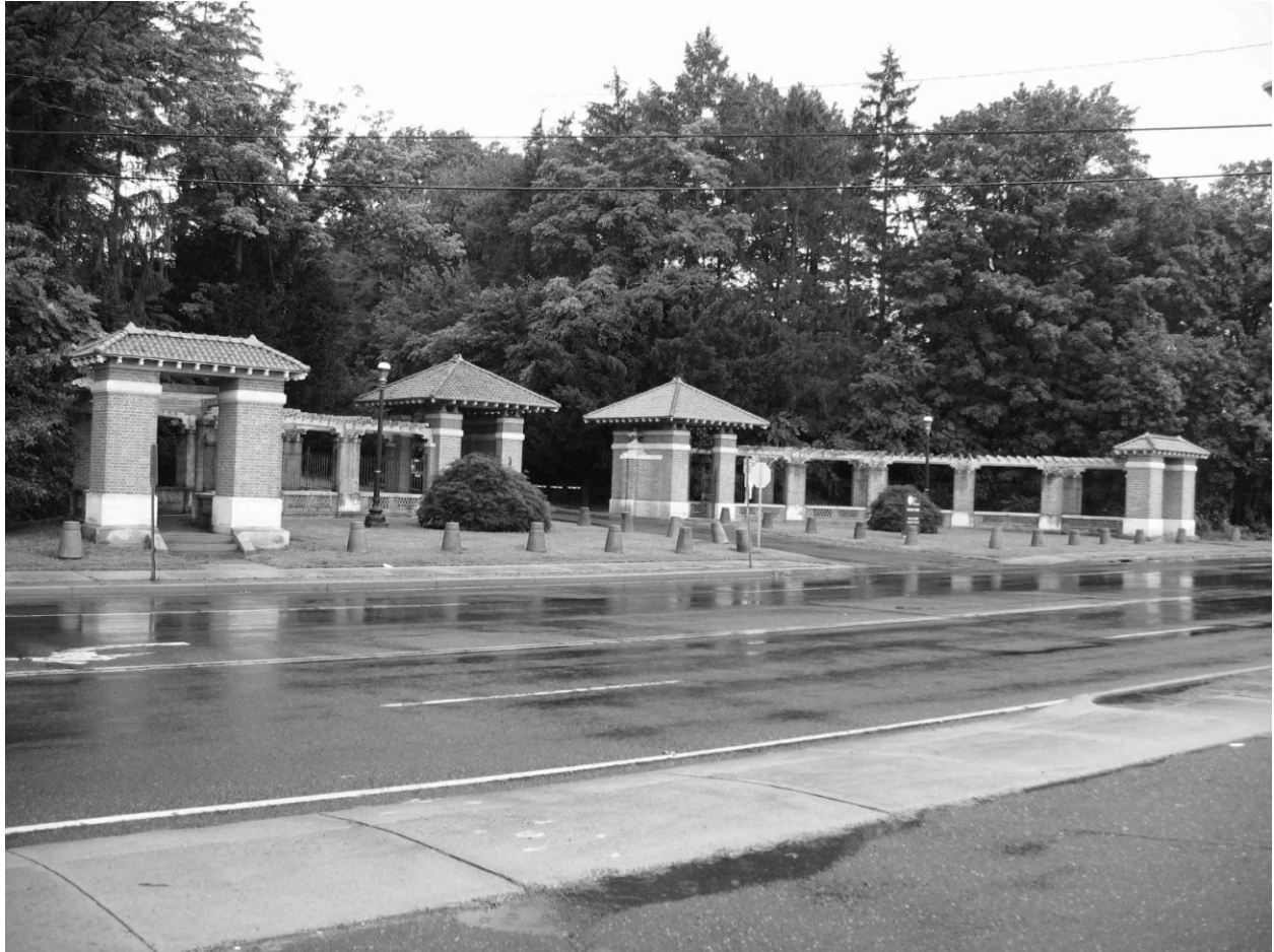
Photograph 32 of 38 Windsor Street gateway Camera facing northwest
