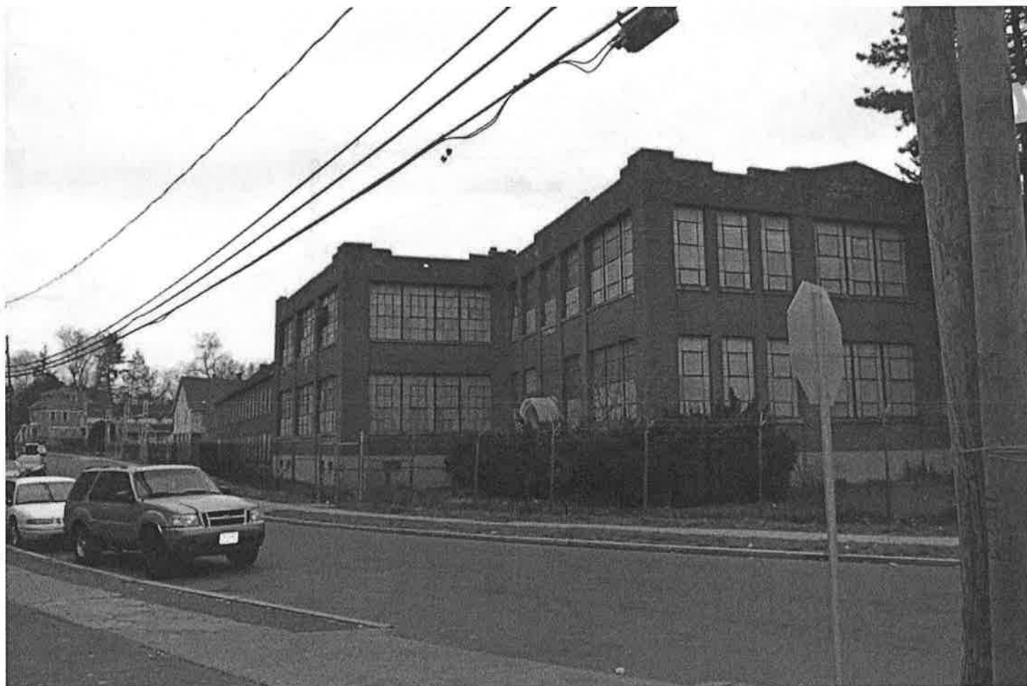
South (front) and west (side) elevations of factory from Love Lane, showing 1929 block with side ell. Camera facing northeast. Photograph 6 of 18.
