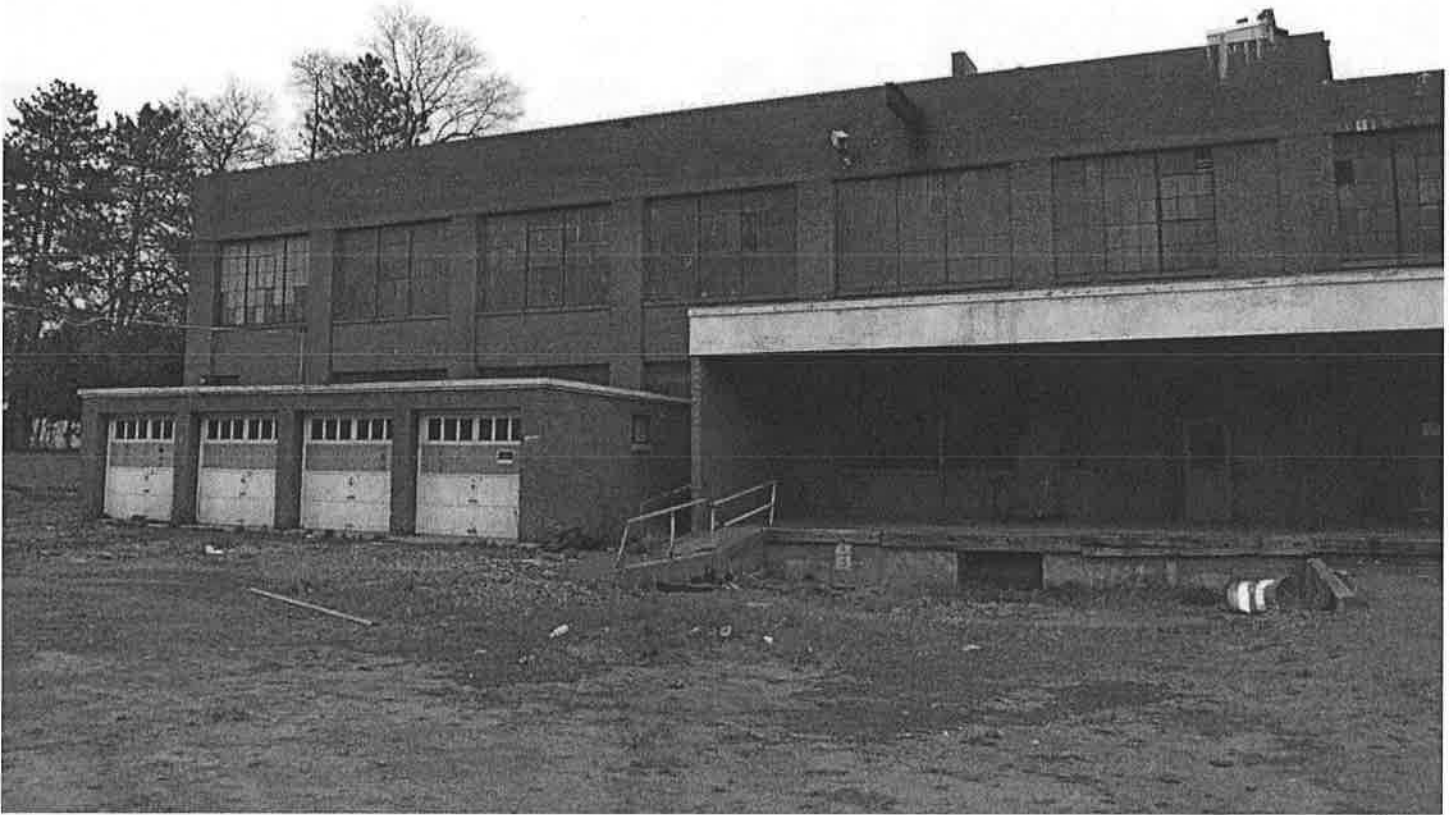
West (front) and south (side) elevations of 1941 garage from Love Lane, 1948 block at rear. Camera facing northeast. Photograph 17 of 18.
