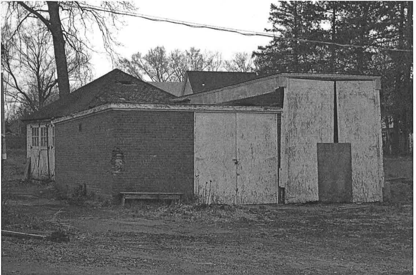
South (front) and north (side) elevations of c. 1960 and c. 1970 storage buildings from Love Lane. Camera facing northeast. Photograph 18 of 18.
