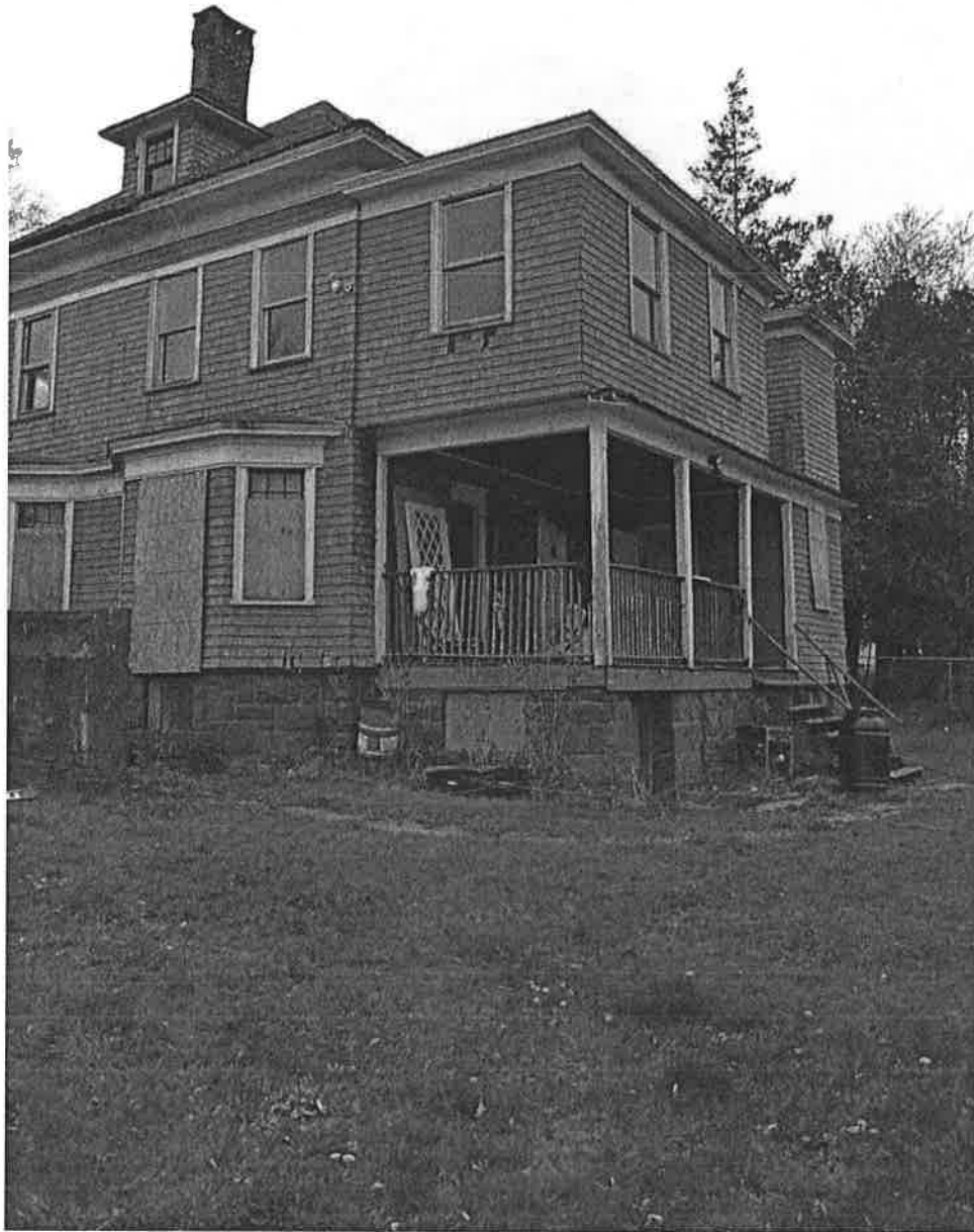
East (rear) and south (side) elevations of 1914 Swift house from interior of property. Camera facing northwest. Photograph 15 of 18.
