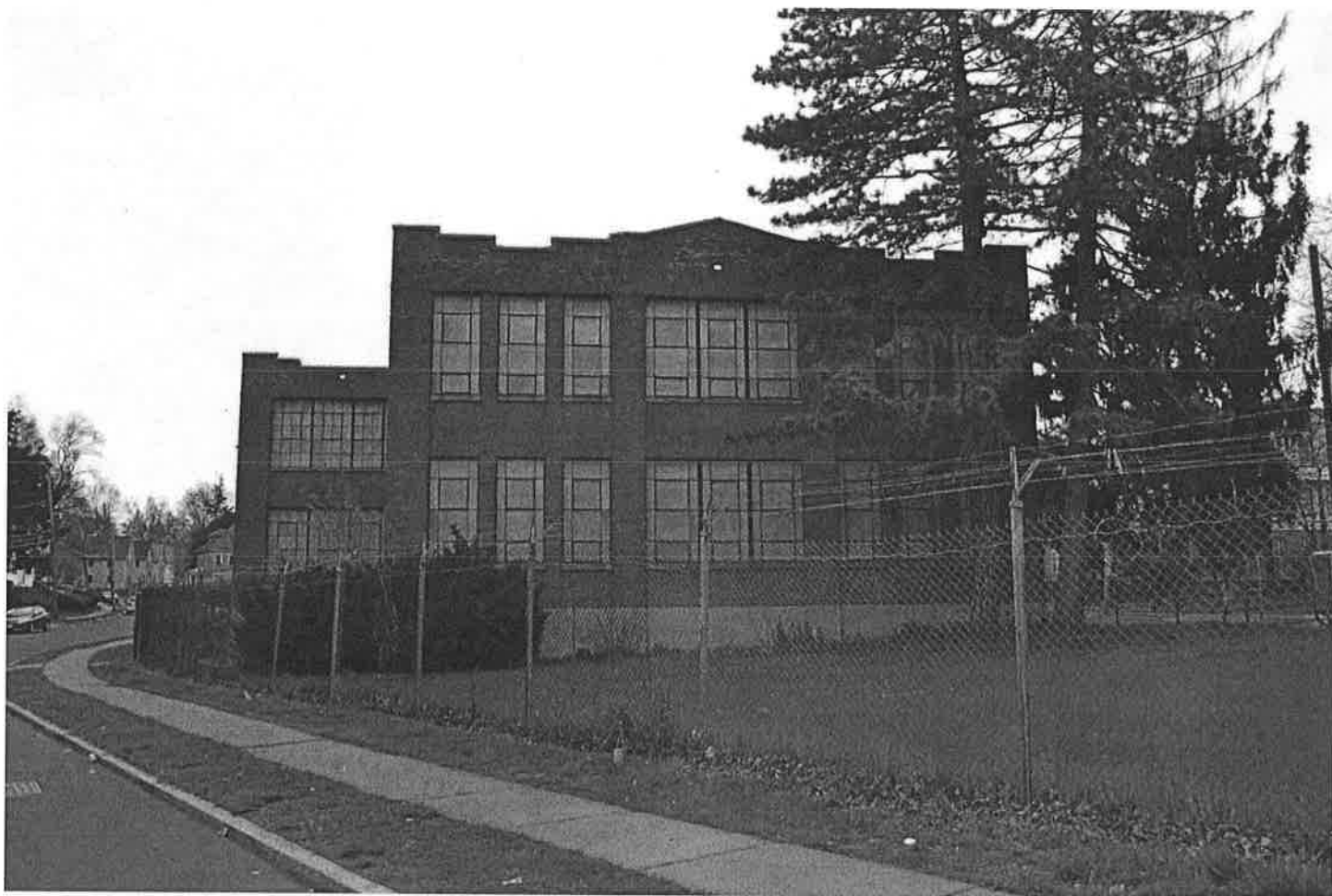
South (front) elevation of factory from Love Lane, showing 1929 block with side ell. Camera facing north. Photograph 5 of 18.
