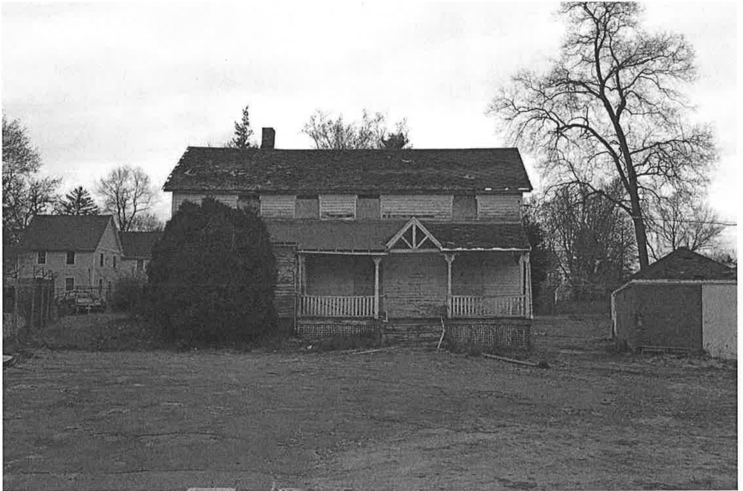
South (front) elevation of Swift homestead (c. 1887) from Love Lane. Camera facing north. Photograph 10 of 18.
