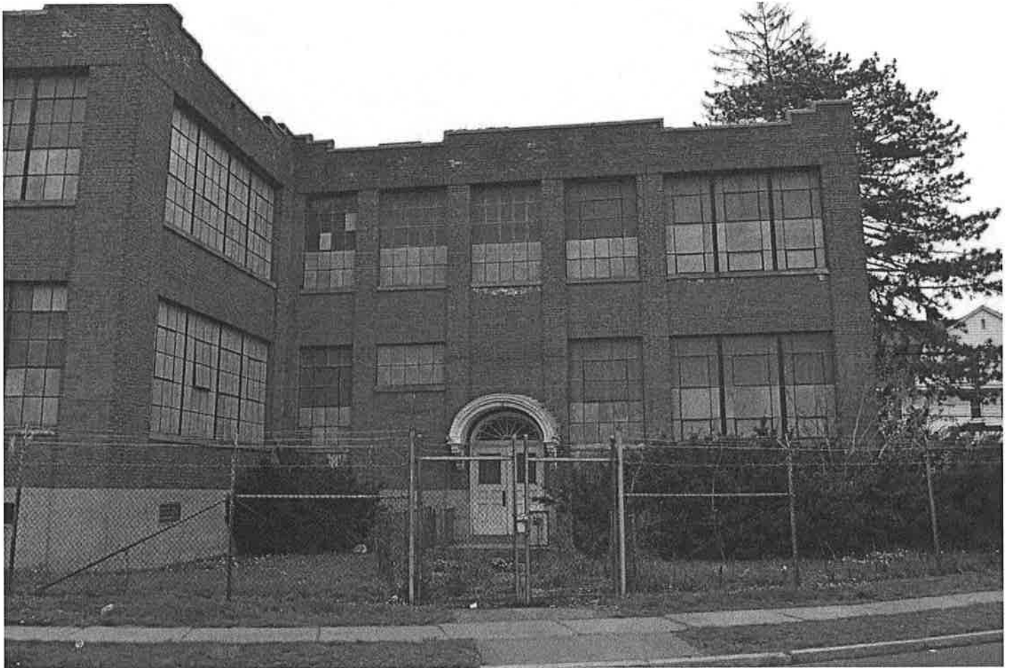
West (side) elevation of factory from Love Lane, showing primary entry in 1929 block. Camera facing east. Photograph 8 of 18.
